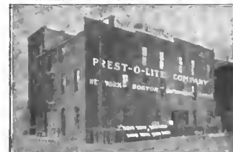
INDIANAPOLIS PLANT NO. 1
